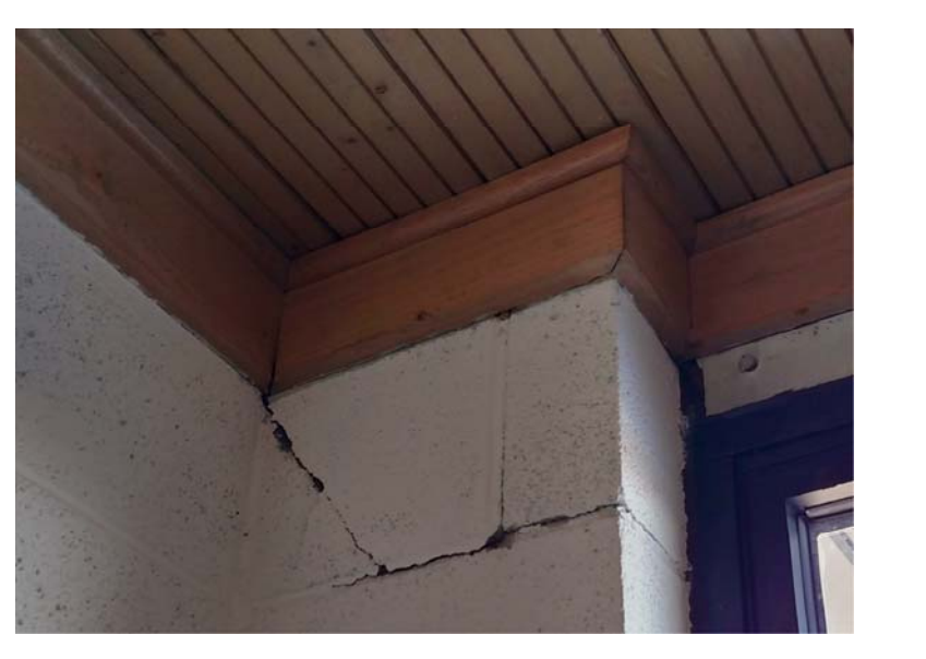
(1A) ELEVATION SCALE: N.T.S. NORTHWEST CORNER OF STORAGE ROOM 129
