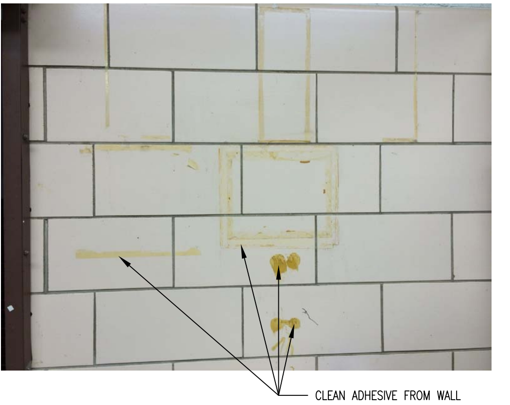
(5C) ELEVATION SCALE: N.T.S. CLEAN ADHESIVE FROM WALL
