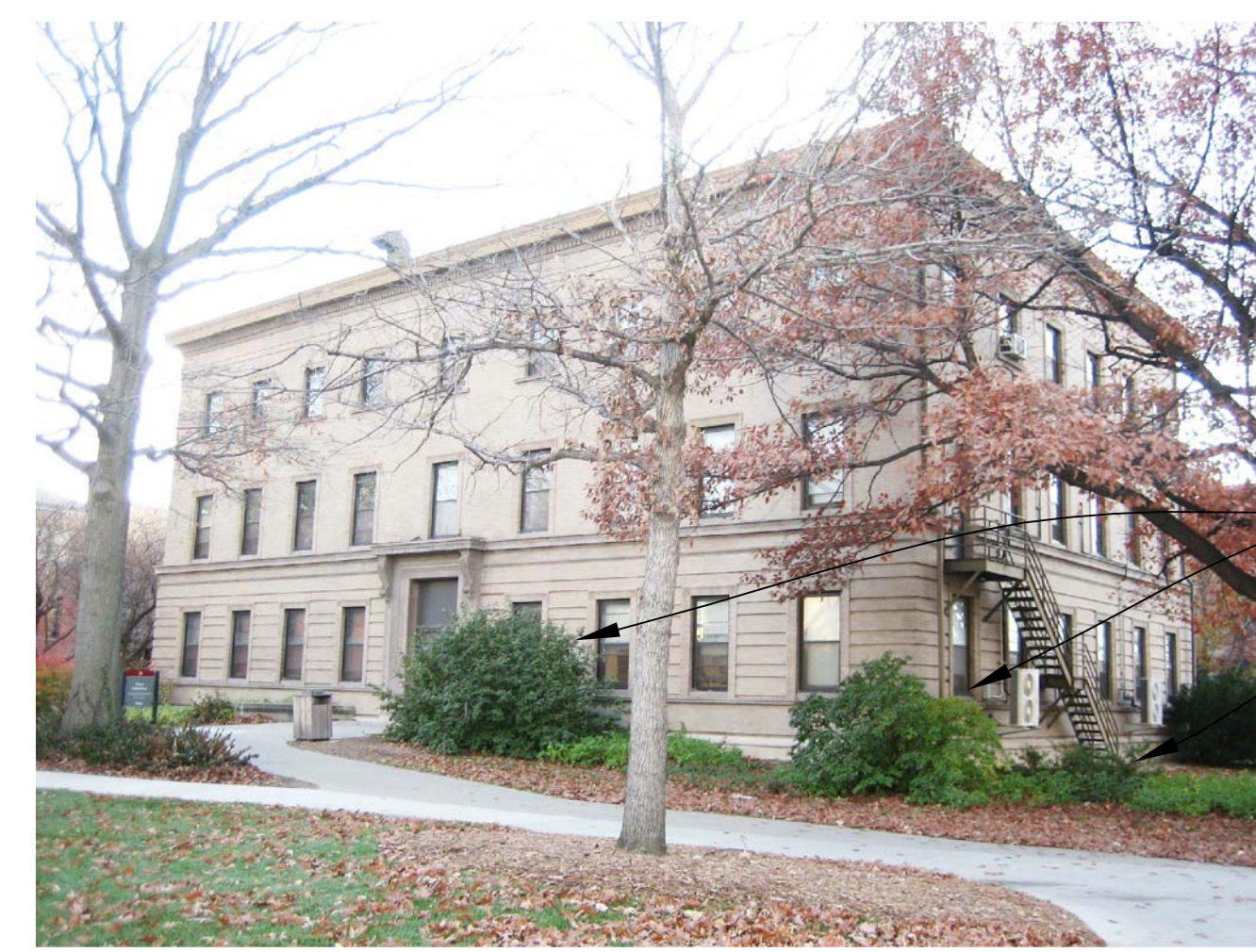
1 PHOTO- NORTHEAST ELEVATION WITH ENTRY DOOR SCALE: NONE
