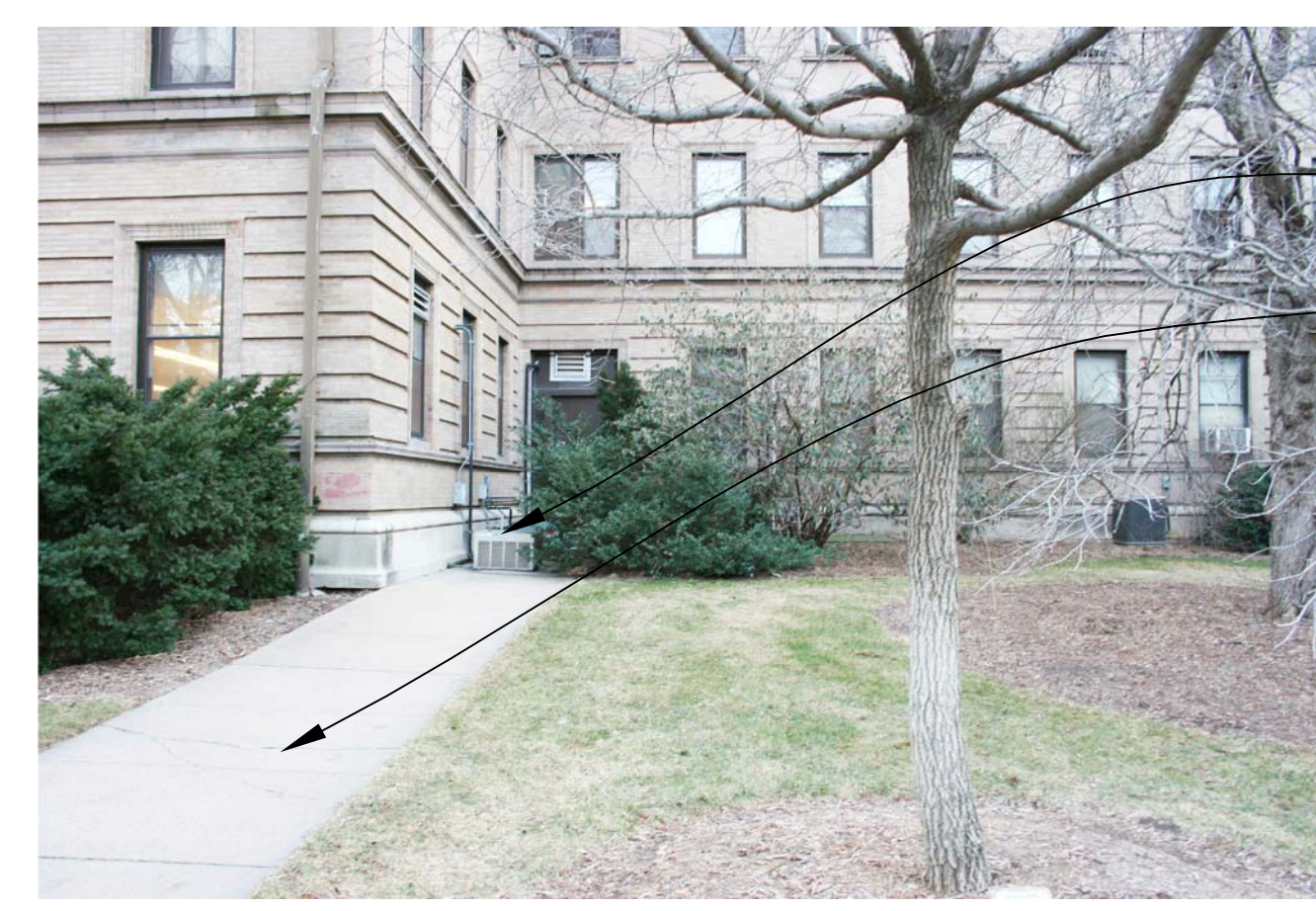
2 PHOTO- NORTH ELEVATION WITH SIDEWALK SCALE: NONE
