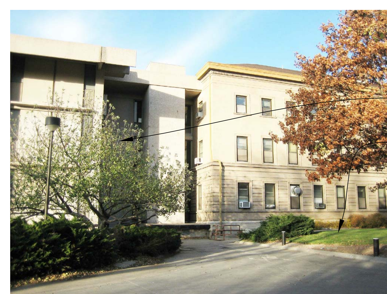
3 PHOTO- SOUTHWEST ELEVATION AT DOCK SCALE: NONE
