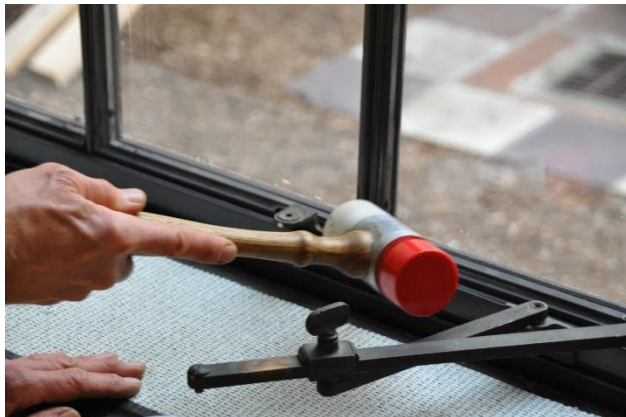
Figure 33 - The brass hardware being gently adjusted for proper operation.
