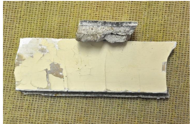
Figure 22 - A portion of the plaster that was removed from the left jamb to facilitate removal of the subframe.
