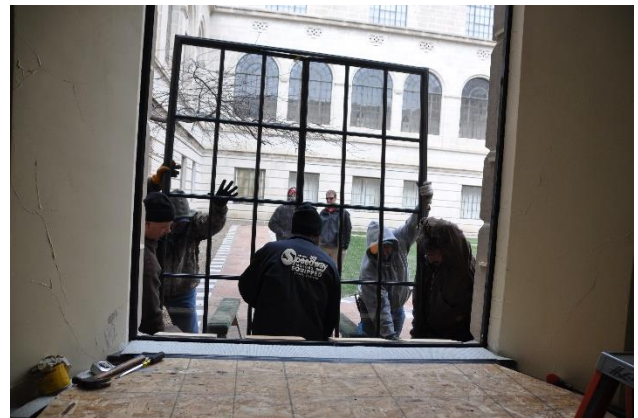
Figure 31 - The sash and frame being hoisted into place.
