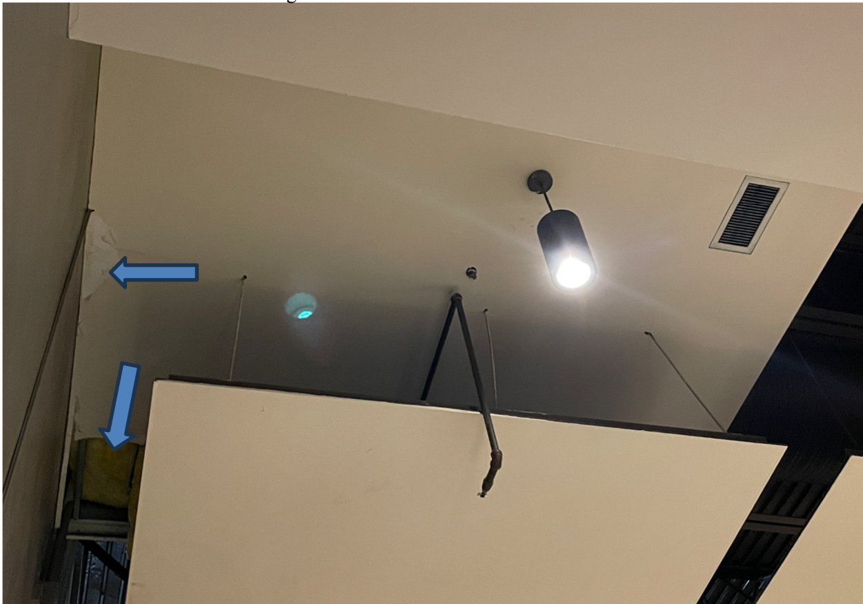
Photo “A” Patch ceiling in Auditorium (repair water damaged area and replace missing gwb in ceiling)
