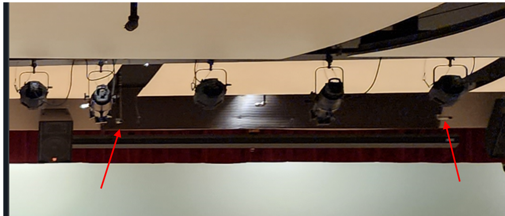
Photo “C” Remove identical pipe on south side of speaker cloth.
