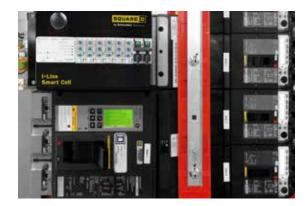
The modular I-Line Smart Cell enables value-added solutions in I-Line panelboards in a variety of combinations. The space-saving unit fits into the I-Line bus in place of a breaker, and allows the I-Line panelboard to be transformed into a digital communication or metered electrical distribution solution.
