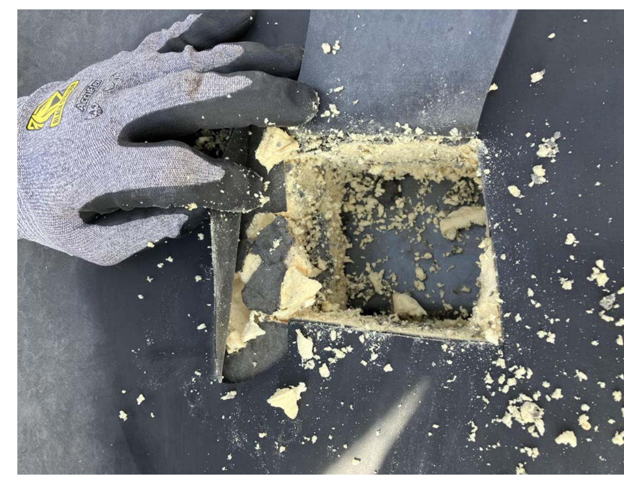
5 INVESTIGATIVE ROOF CORE 2 D1.0
