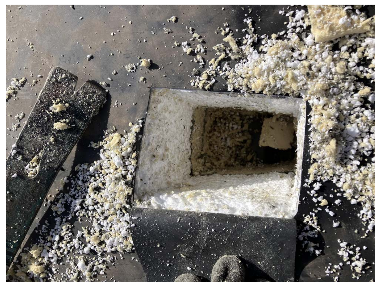
3 INVESTIGATIVE ROOF CORE 1 D1.0
