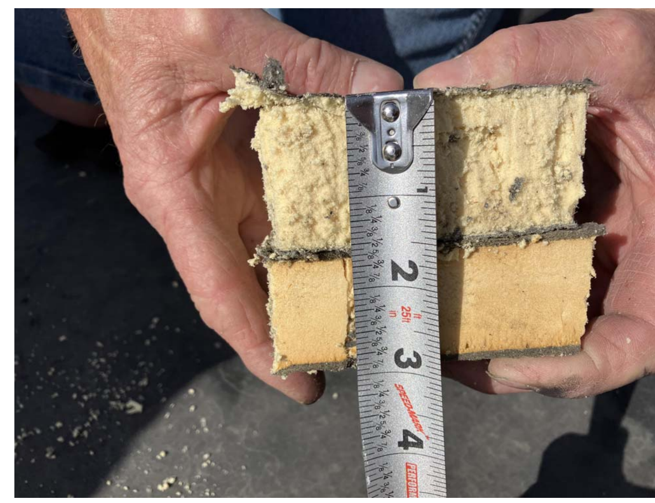
4 INVESTIGATIVE ROOF CORE 2 D1.0
