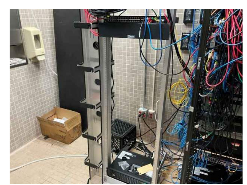
2B PHOTO EXISTING EQUIPMENT ES2.01 SCALE: NOT TO SCALE
